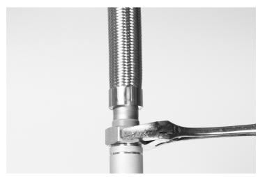
**6.** Bend the flexible hose to achieve the required routing maintaining the minimum bend radius and position the reducer for sprinkler location. When bending the hose allow 65mm of straight hose from the nut, ensure there are no kinks.
