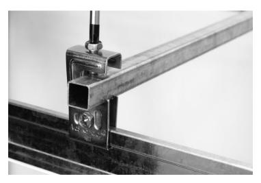
**7.** Slide A2 type centre bracket onto the square bar, mount the outlet reducer through the centre bracket and lightly tighten the nut. Adjust location of the centre bracket and the side brackets until desired location of the outlet reducer is achieved. Firmly secure the side brackets by tightening the screws to a torque of 5 Nm/4 ft-lbs.
